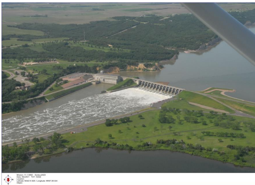
Figure 1.3: Missouri River, Gavins Point Dam and Reservoir (Tretbar, 2011)
